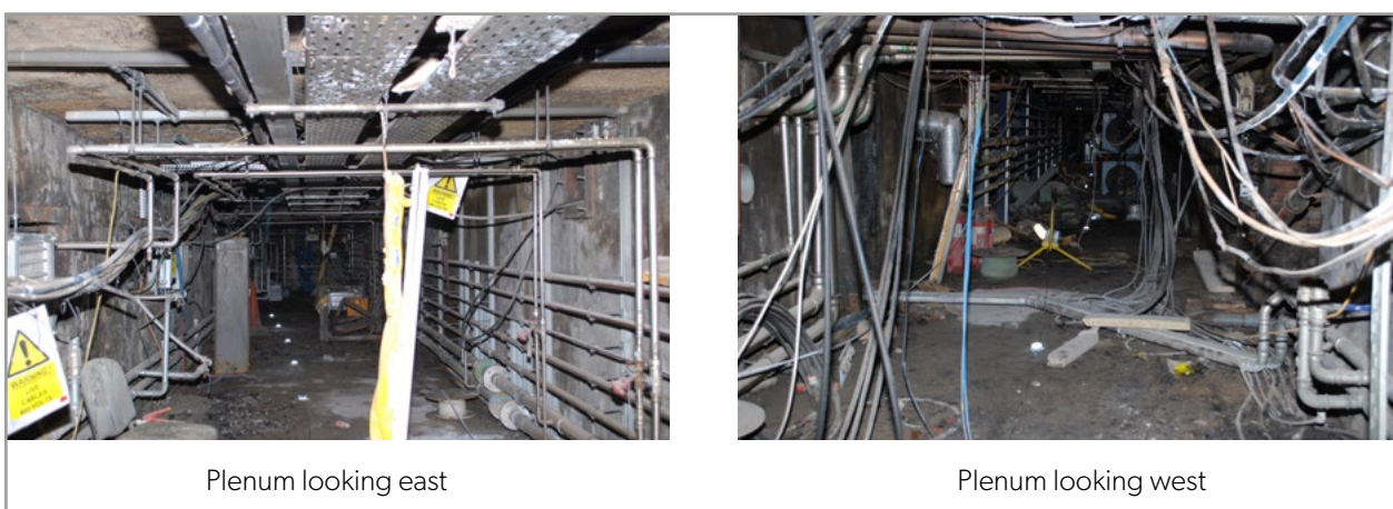
Figure 18 – Plenum below level 2
