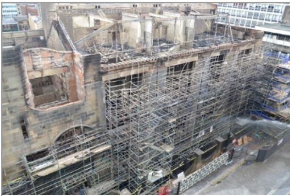
North Elevation, west end Renfrew Street Scott Street corner
