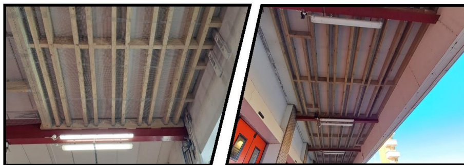
RAAC Remediation at Galashiels
