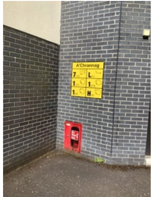
Figure 4: Indicator plate in place on the block shown in figure 2 Source: HMFSI
