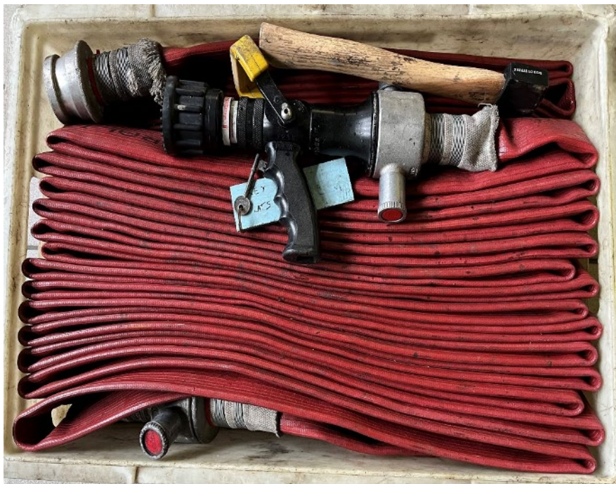
Figure 5: Legacy high rise equipment box in SFRS (with flaked hose)
