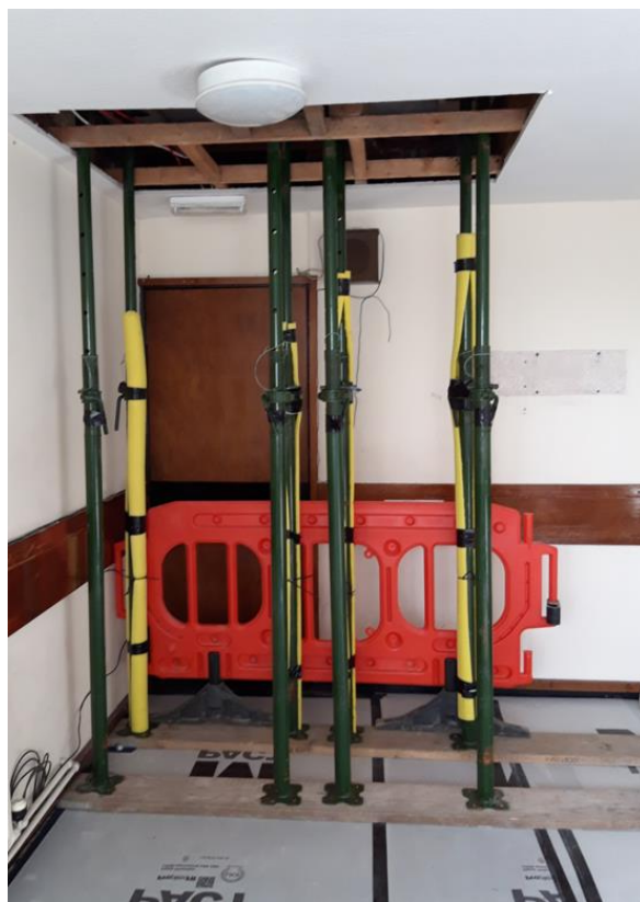
Steel Props at RAAC roofing sites
