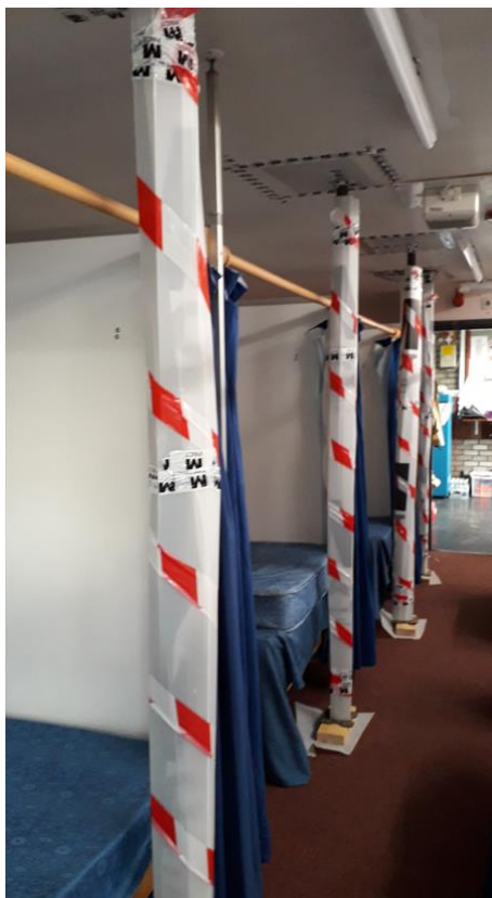
Steel Props at RAAC roofing sites
