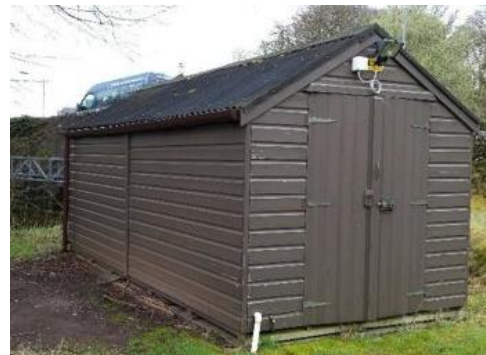
Colintraive Fire Station
