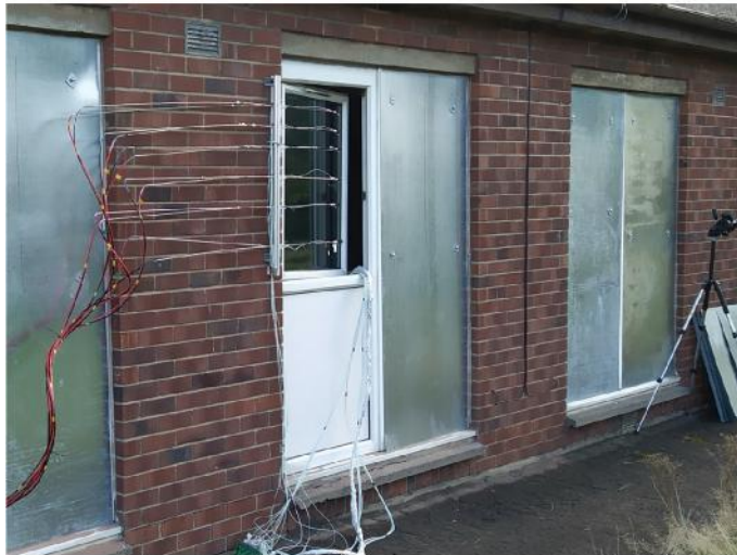
Figure 6 The position of the flow measurements in Room 1.
