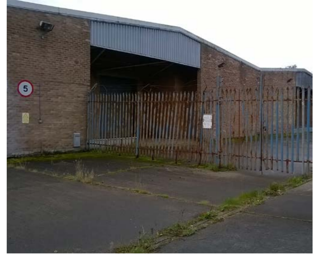
Building As Existing
