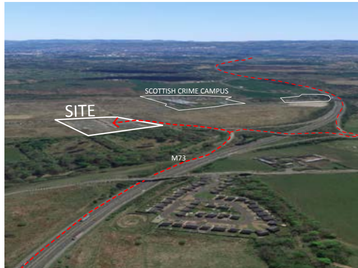
Plot 1A West looking South
