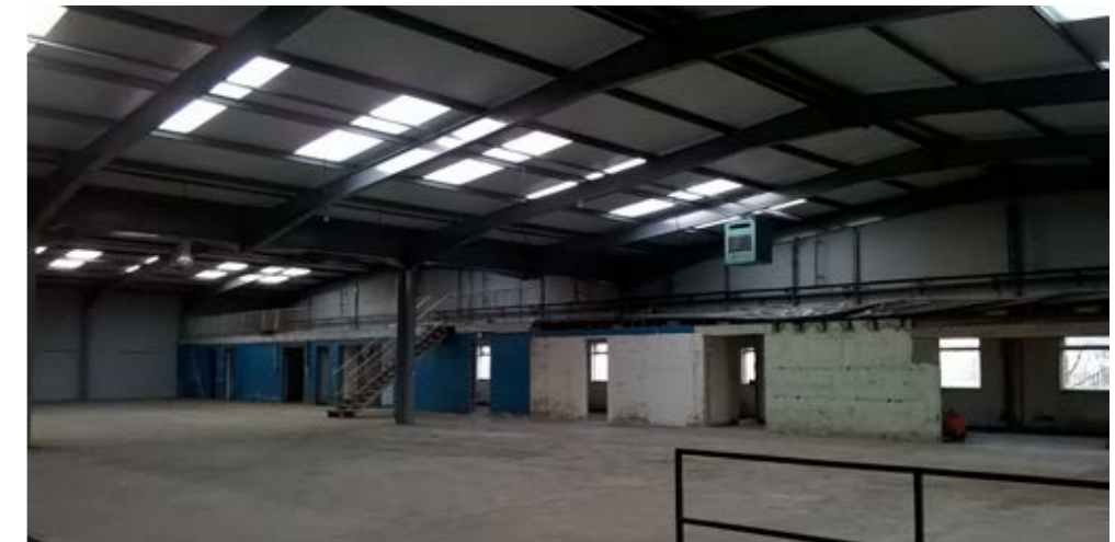
Building As Existing- Warehouse Interior
