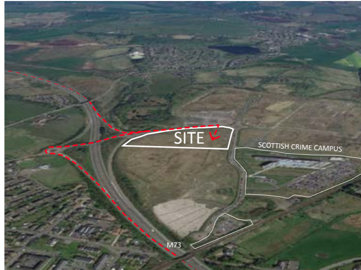
Plot 3 looking North East
