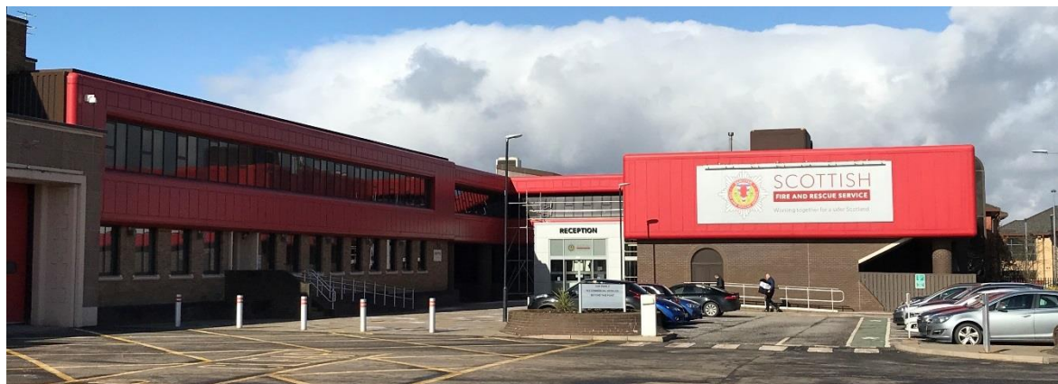
Main entrance and reception, Bothwell Road, Hamilton
