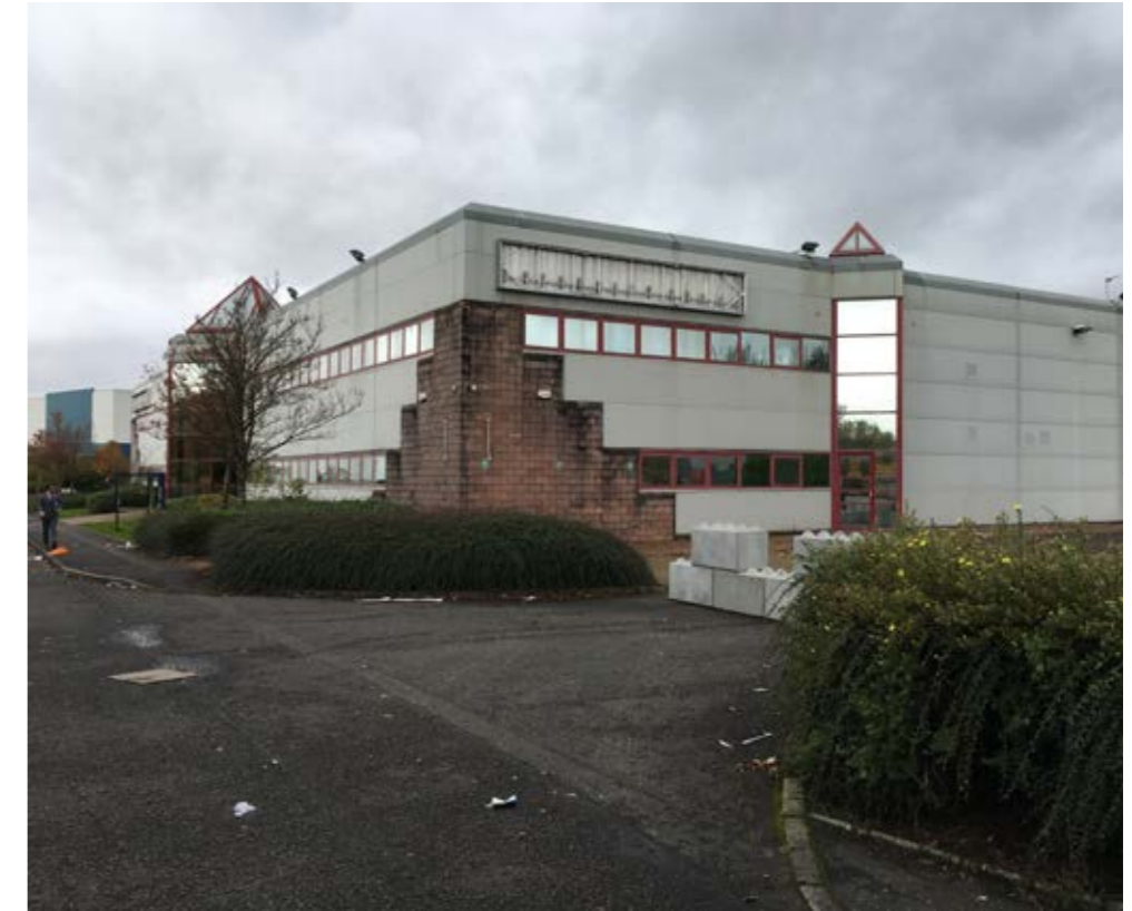
Building As Existing
