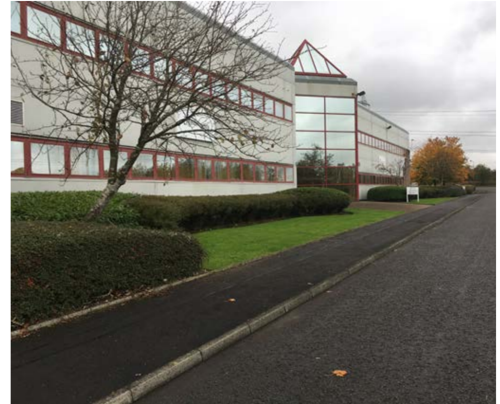
Building As Existing
