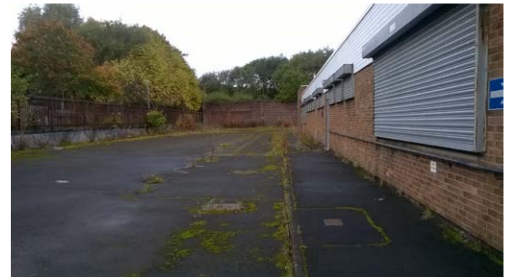
Building As Existing- Rear Yard
