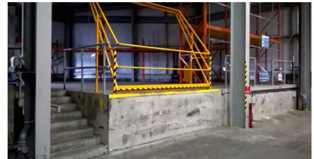
Building As Existing- Warehouse Interior
